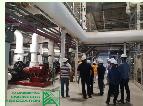
The utilities facility at the airport
