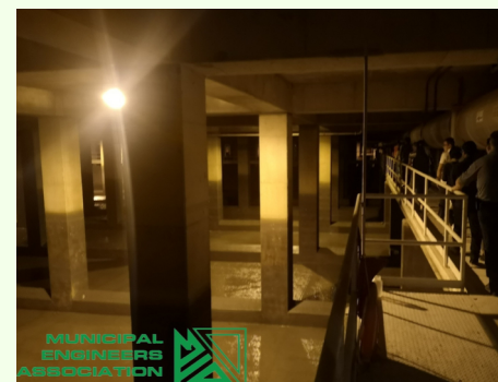
Underground storm water facility with 44 Million Liters of capacity
